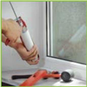
Air Sealing & Insulation
